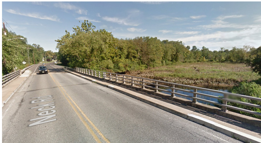
Figure 3: Assiscunk Creek Bridge at Neck Road
